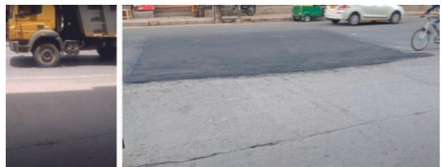
In HSR Layout, in the KEB Junction, a patch of road was dug up for the Metro line by the Bengaluru Metro Rail Corporation Limited (BMRC) to lay the power cable line from Karnataka Power Transmission Corporation Limited (KPTCL). Once the cabling work was complete, the road was restored by tarring the patch. We sincerely thank the BMRC team for their support.
